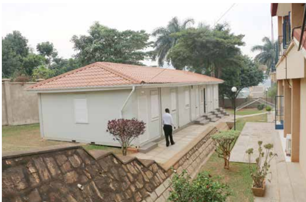
Human Rights House Annex constructed in 2015
