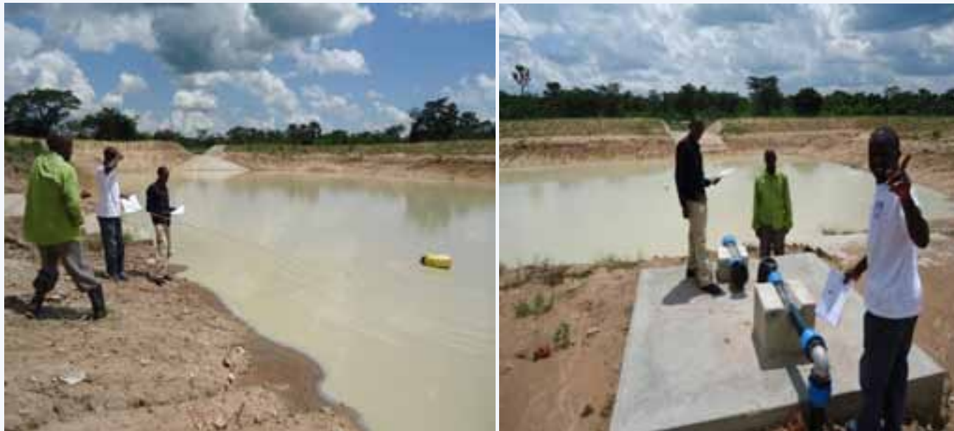
Community monitors examining water pipes at Kakabala valley dam in Dwaniro sub-county, Kiboga district, 22 nd May 2013.
